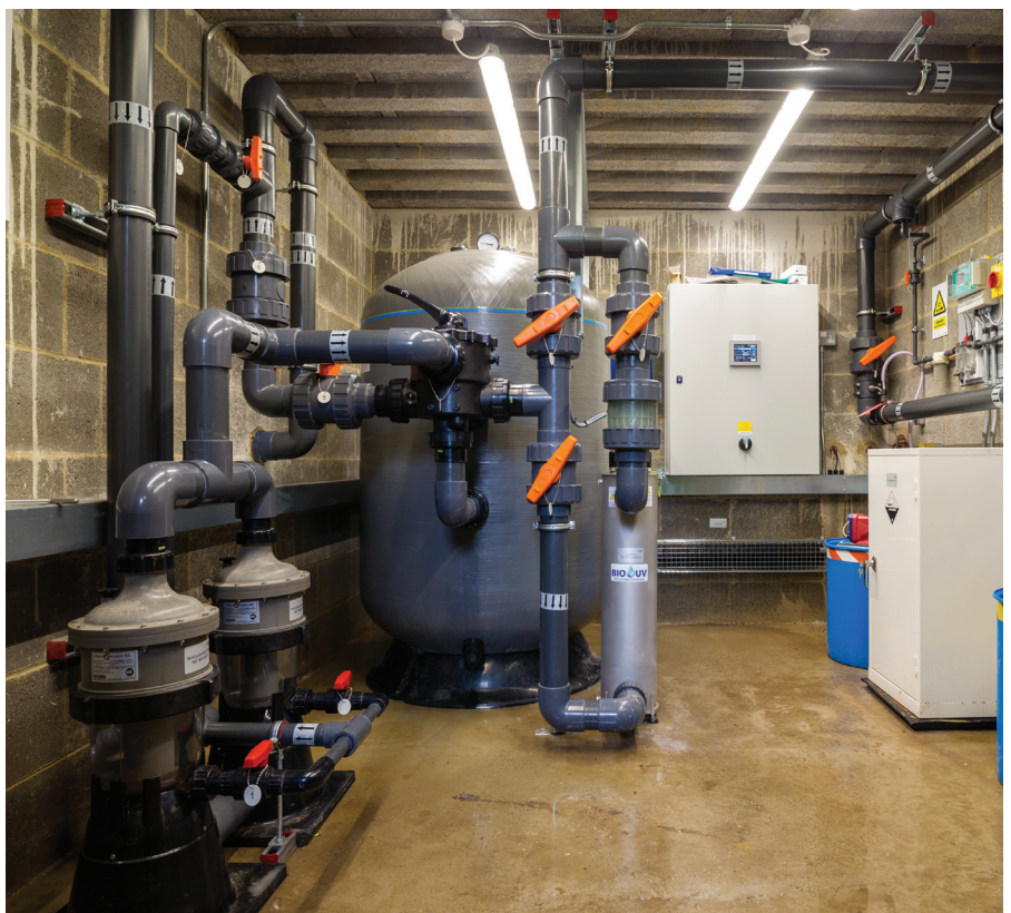
Waterco's commercial-grade water treatment products to ensure water quality complies with PWTAG guidelines and materials withstand the corrosive environment.
