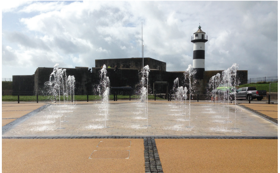
Fountains Direct managing director Nick Roberts proposed a multi-jet dry plaza fountain centrally placed within the existing space.
