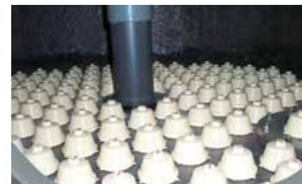
Nozzle Plate under drain system
