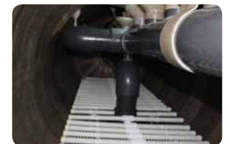
Internal plumbing & laterals
