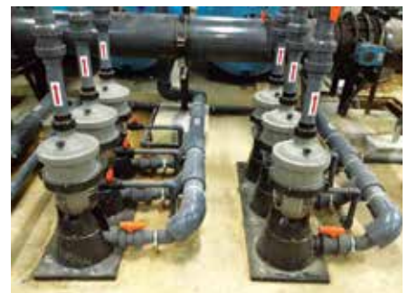
18 MultiCyclones are installed to minimise filter maintenance and save water.
