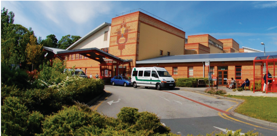
Southport and Ormskirk Hospital offers a comprehensive, individually-tailored and family-oriented approach to spinal cord injury treatment.
