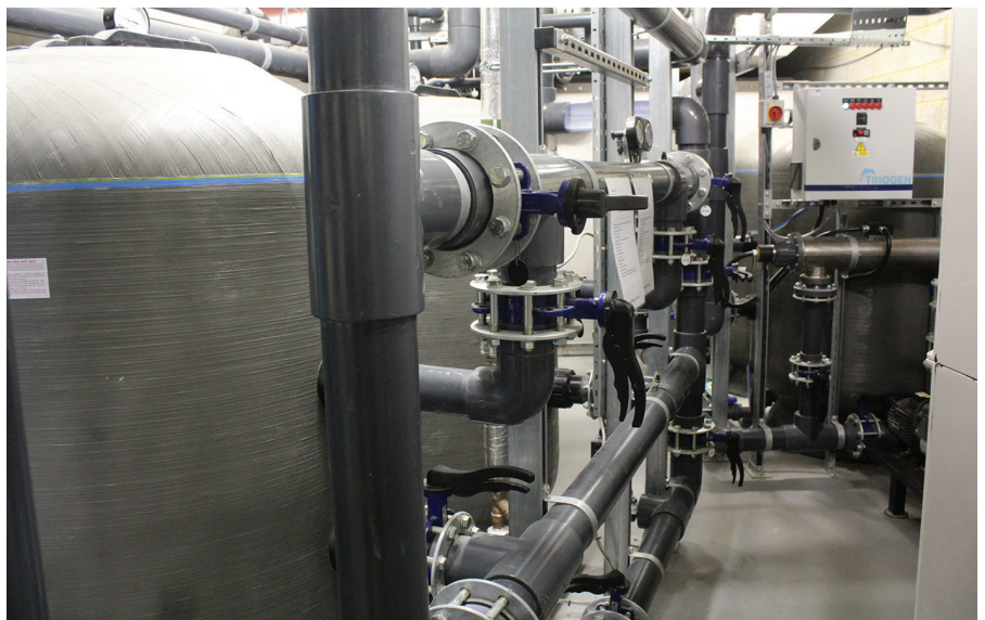
Manufactured from the highest grade of non-corrosive materials and employing the latest in fibreglass winding technology, Micron filters are designed and built for many years of trouble-free operation.
