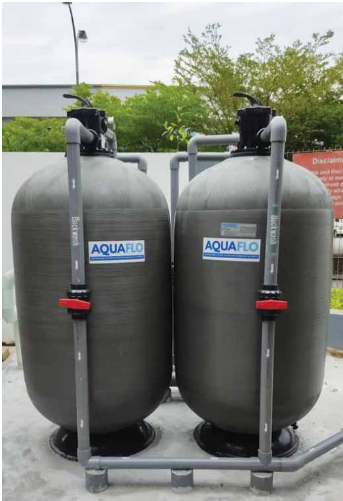
Two units of AquaFlo Centralised Water Filters (model: AQ900X) were installed to cater to the filtration needs of Senai Garden
