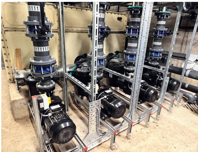
Four Waterco Hydrostar Plus pumps draw water from the main reservoir and back to the feature.
