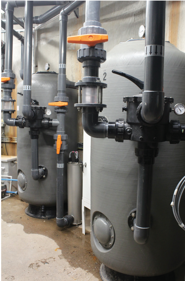
Micron SMDD900 commercial media filters and re-entering the feature via the main reservoir.
