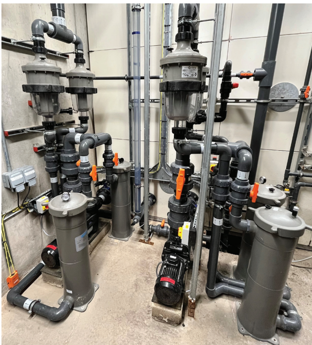
2 x C75 bag filters and double manifold MC16 centrifugal filtration units.
