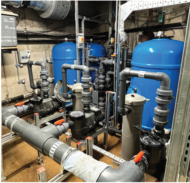
Hydrostorm Plus pumps and C75 Trimline bag filters ensure it is filtered to the very highest quality.
