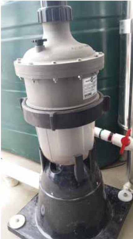
MultiCyclone is a pre-filtration device that works on the basis of centrifugal water filtration and is designed with no moving parts and no filter media to clean or replace.
