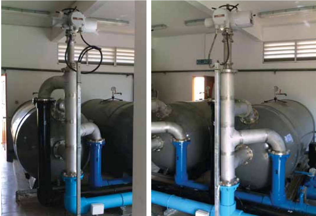
◀ Two Micron M5000 (horizontal) filters and three SMD1400 (side mount) filters.
