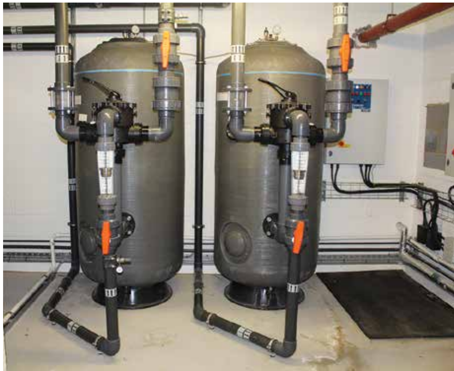
▲ The main filtration for the pedestal water clock feature is operated by a separate plantroom to the communal courtyard feature. Water is drawn from a holding tank and comprises of 2 x Micron SMDD900 commercial filters complete with 3" MPV's and 2 x Hydrostorm Plus 3HP commercial pumps that are plumbed in conjunction with 2 x MC16 multicyclones for sediment removal. Also 2 x Hydrostar 7HP commercial pumps are installed for the overflow effect and circulation.
